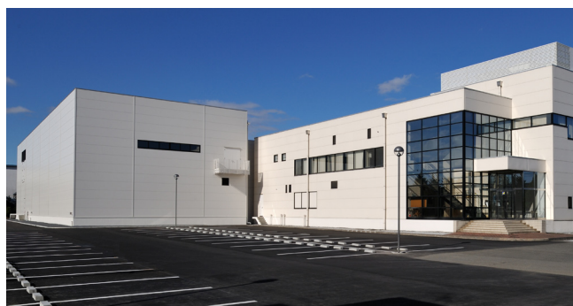
Nipro Patch Co., Ltd. Hanyu Plant
