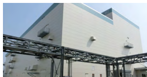
New building construction for hormone drugs
