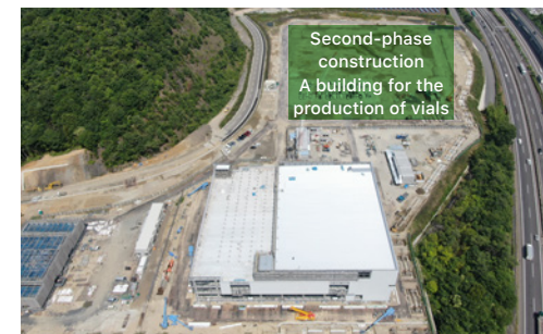
Omi Plant, Nipro Pharma Corporation under construction
