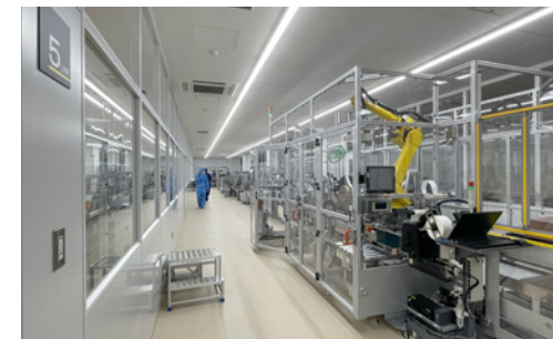
PTP packaging line under construction
