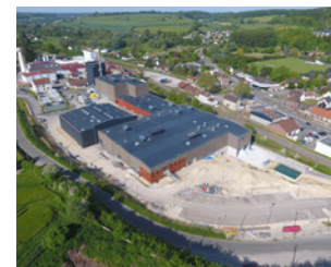
Overall view of the new glass tubing facility in Aumale, France
